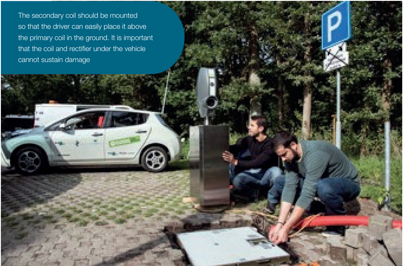
Figure 18: Installation of the wireless charger in Rotterdam
