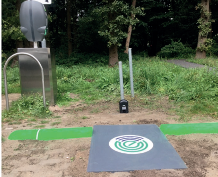
Figure 6: Wireless charging system as implemented in Rotterdam
