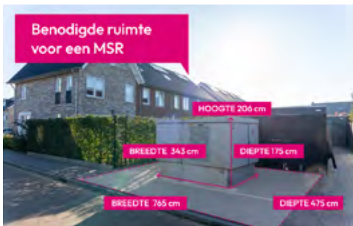
Fig 5. Afmetingen MSR Enexis (206 H x 765 B x 475 D (cm), 36 m 2 )
